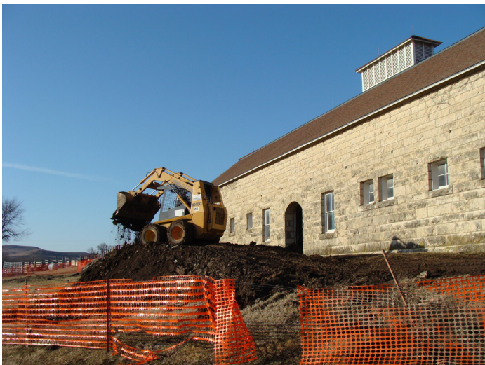
Renovation of the barn
