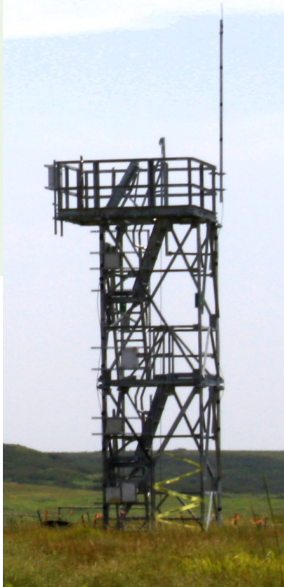
NEON core tower on Konza, during construction in 2014
